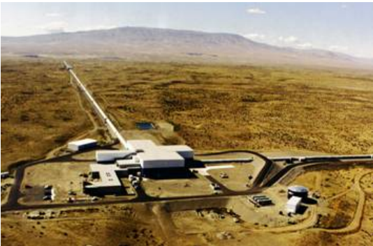
Figure XX: Photographs of the LIGO Observatories in Livingston, LA (right) and in Hanford, WA (left). The Hanford facility comprises two co-located interferometers, sharing the same vacuum enclosure but otherwise independent, with 2 and 4 km baselines. Credits – LIGO lab
