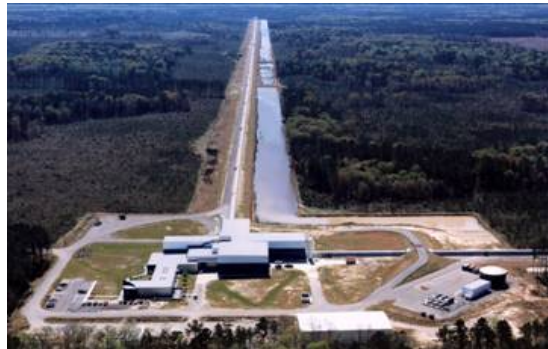
Figure XX: Photographs of the LIGO Observatories in Livingston, LA (right) and in Hanford, WA (left). The Hanford facility comprises two co-located interferometers, sharing the same vacuum enclosure but otherwise independent, with 2 and 4 km baselines. Credits – LIGO lab
